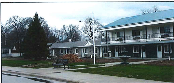
Figure 1 Blue Haven Apartments in Amherstburg, Ontario
